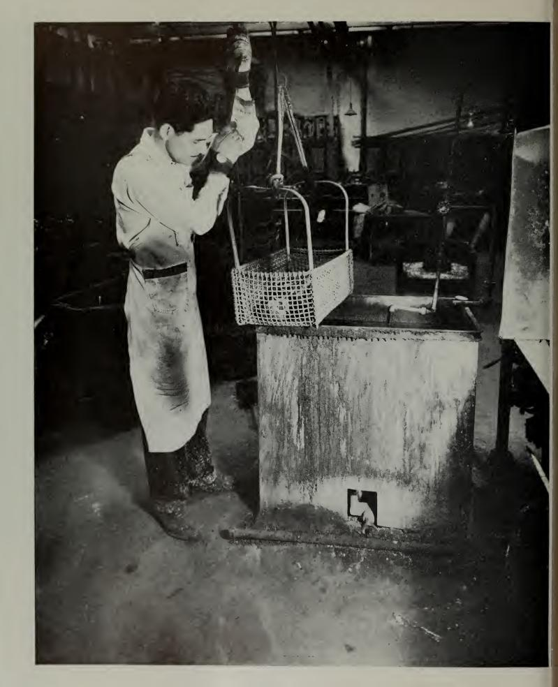
Then the rods are dipped into an oakite tank as shown above for cleaning.
